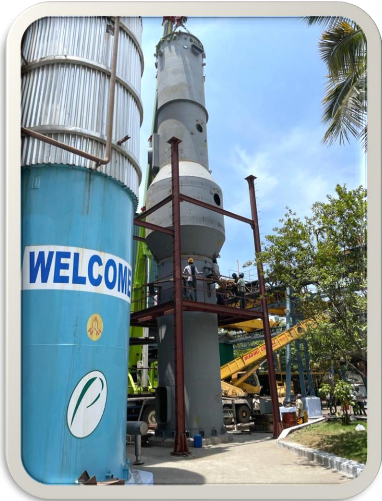
2500M2 Falling Film Evaporator Installation
